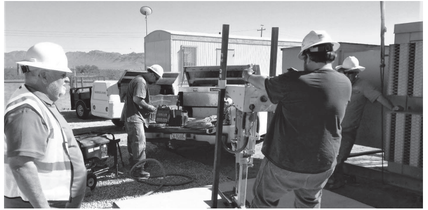
Dan M. Offret watches the installation of an auxiliary power generator at the Metro Southwest – Diablo Village No. 2 well in 2015. 💧
