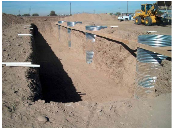
Photo 2 - View of one of two plots that will be used to evaluate growing halophytes to manage concentrate produced during RO treatment. Each plot is lined with 40-mil HDPE geomembrane. The 6-foot diameter manholes will be used to monitor irrigation water applied to the plants.
