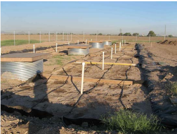
Photo 7 – The finished product-lined plots awaiting irrigation piping and planting.
