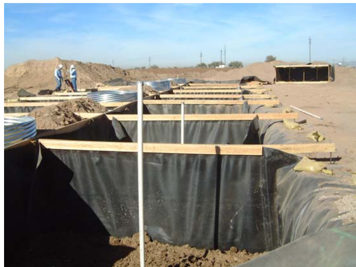
Photo 4 – The lined plots were divided up into sections to monitor water uptake using a variety of plant species.
