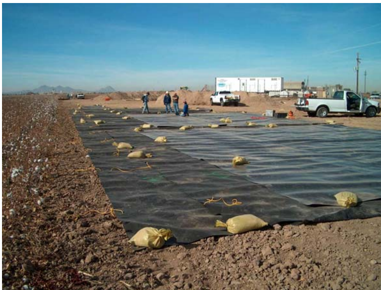
Photo 1 – HDPE liner fabrication for the halophyte plots (40 mils) and the SSF filter cells (60 mils). Over 9,000 feet of liner were fabricated on site for use in the halophyte plots and slowsand filters.
